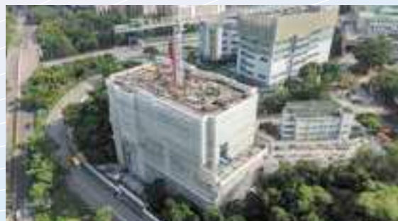
擴建計劃第一期新大樓的上蓋工程現正進行，預計2027年底落成，2028年第二季投入服務 Superstructure works for the new "Hospice Care Block" are now in progress. The building work is scheduled for completion by the end of 2027, with service commissioning in the second quarter of 2028.
